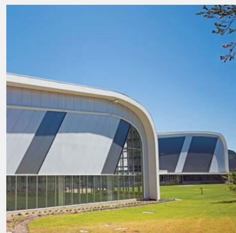
It should be noted that MW does not offer transparency, only translucency. This produces the diffused light where objects behind the panels will appear blurry. This is often an advantage in public spaces where the softer, diffused light is more comfortable. Another benefit is the fact that any defects, stains, bird droppings, etc., are less visible.
