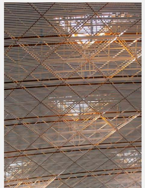
As an example of MW's versatility in design, triangular-shaped "dragon scale" skylights adorn the rooftop of Beijing International Airport's Terminal 3. In all, 45,000 square meters of Palram's 25 mm clear MW create a daylit interior and attractive exterior aesthetic.
